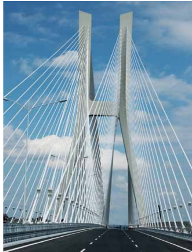
Rędziński Bridge on the Wrocław Motorway Bypass – photo: Marcin Lenar
