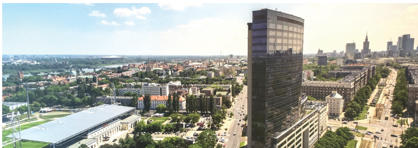
North Gate, DEKA Immobilien
